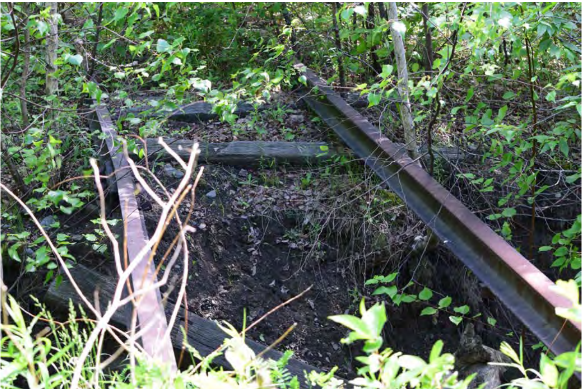
Washout of Pan Am rail bed near Acme Road
