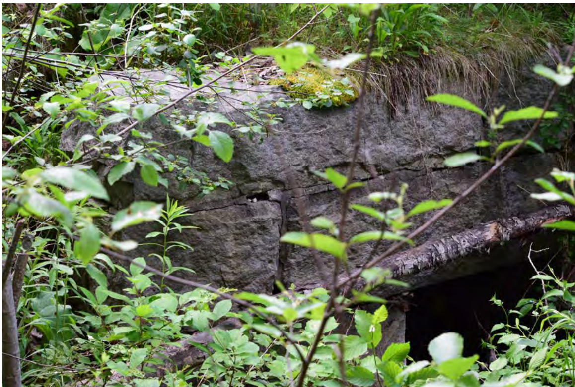
Granite culvert under Pan Am rail bed
