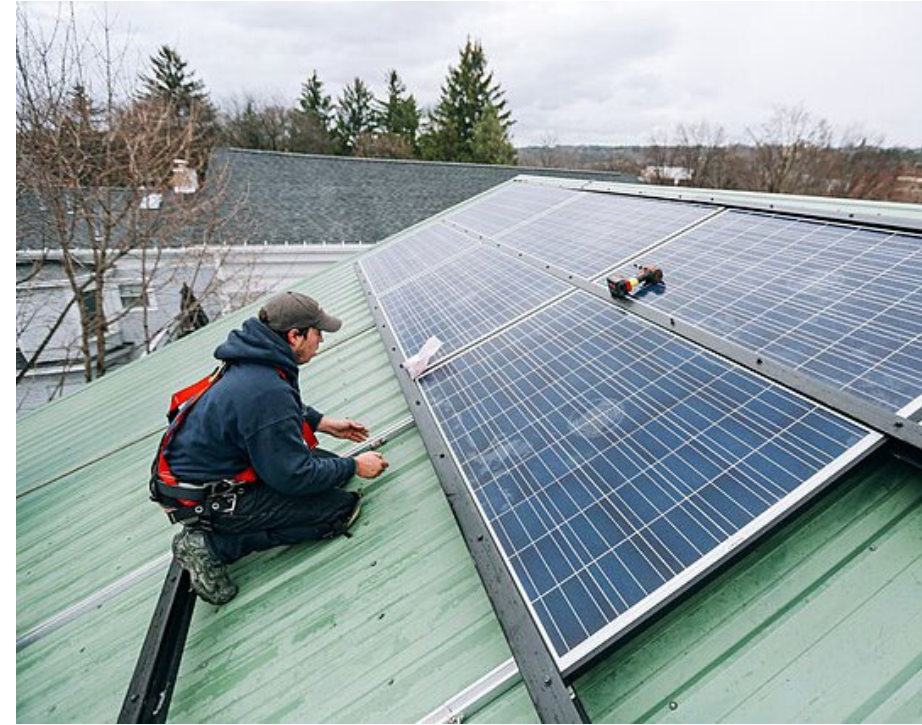
Solar panel installation • Photo by Stephen Yang
