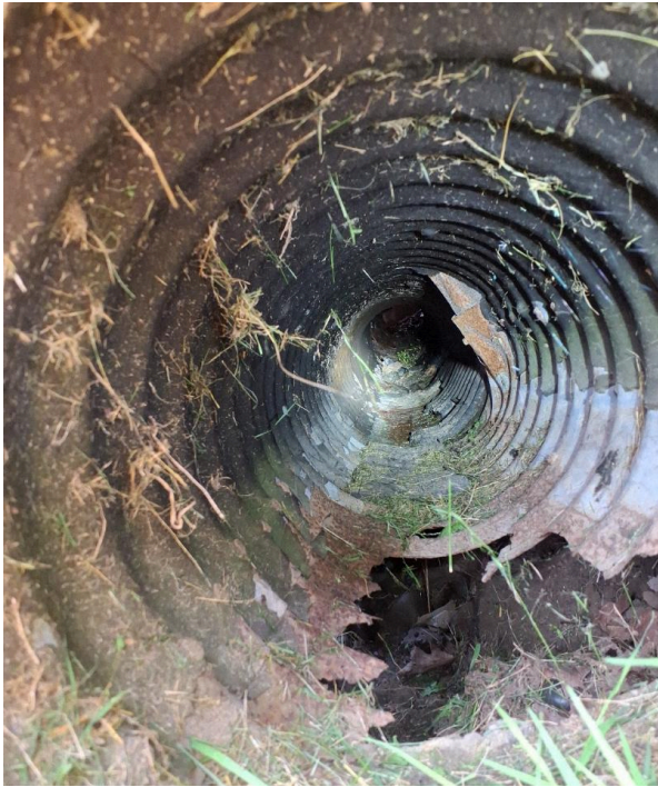
Figure 18: Example of a rusted culvert inspected during the 2025 field season (Culvert ID # 216).
