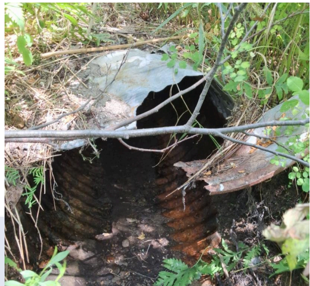
Figure 17: Example of a rusted culvert inspected during the 2025 field season (Culvert ID # 343).
