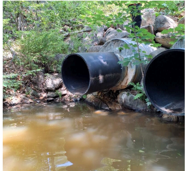
Figure 15: Example of a perched culvert inspected during the 2025 field season (Culvert ID # 1053).
