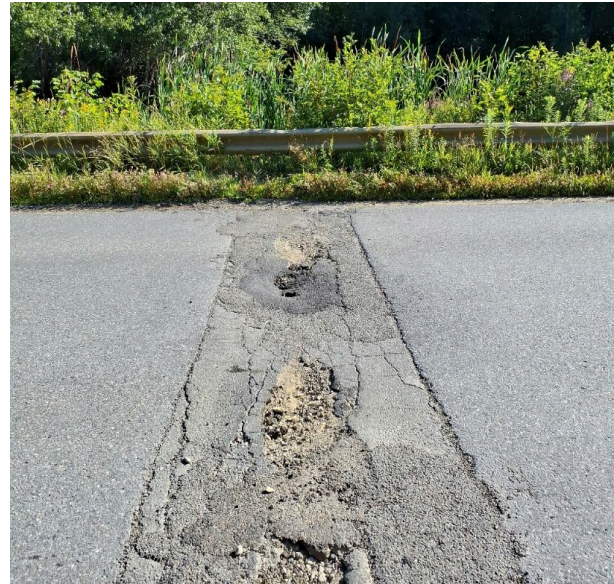
Figure 7: Example of cracking/heaving located at an inspected culvert during the 2025 field season (Culvert ID # 224).
