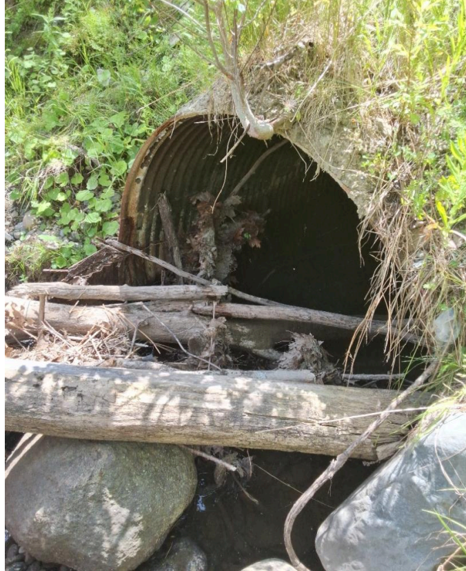
Figure 26: View of a culvert crossing requiring maintenance/replacement that was inspected during the summer of 2025 field assessment (Culvert ID # 8).
