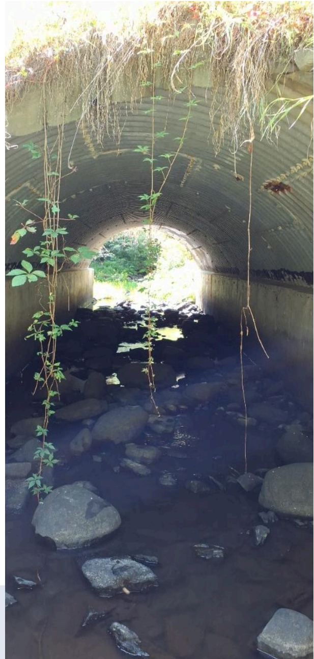
Figure 30: Example of a culvert that includes natural stream substrate (Culvert ID # 1032).
