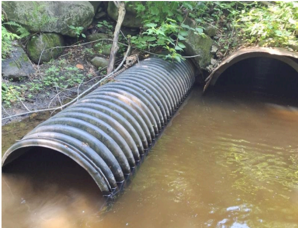
Figure 10: Example of an undersized and submerged culvert inspected during the 2025 field season (Culvert ID # 131).
