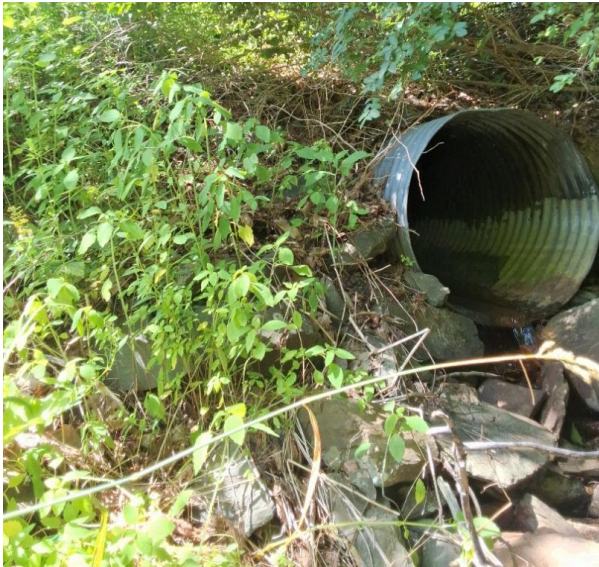
Figure 14: Example of a perched culvert inspected during the 2025 field season (Culvert ID # 78).
