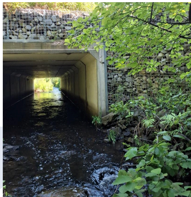
Figure 28: Example of a crossing that includes natural stream substrate (Culvert ID # 289).
