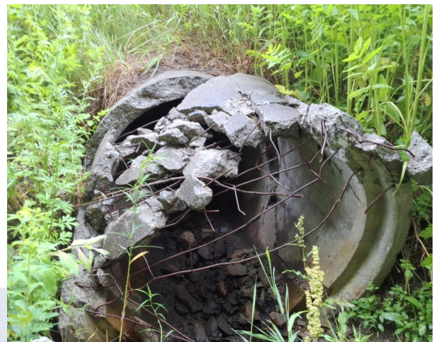
Figure 9: Example of structural failures visible at the inlet/outlet of a culvert inspected during the 2025 field season (Culvert ID # 195).
