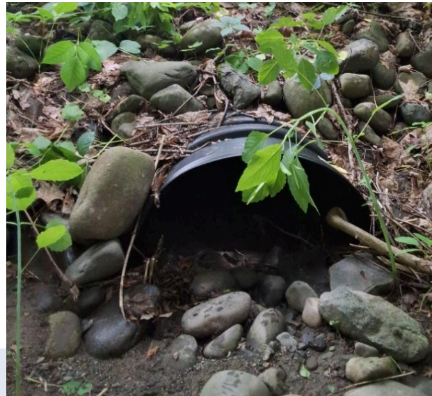
Figure 13: Example of a blocked culvert inspected during the 2025 field season (Culvert ID # 33).
