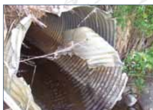
damaged culvert
