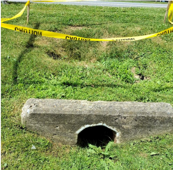
Figure 6: Example of a sinkhole located at an inspected culvert during the 2025 field season (Culvert ID # 216).
