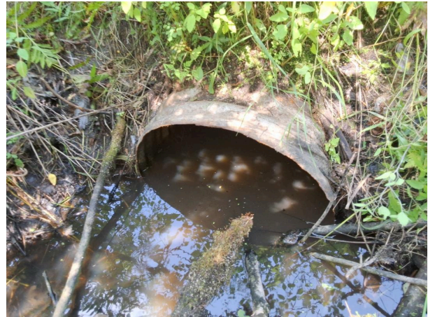
Figure 11: Example of an undersized culvert inspected during the 2025 field season (Culvert ID # 344).
