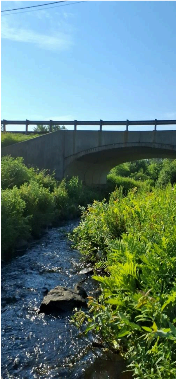
Figure 29: Example of a crossing that spans the stream channel, includes natural stream substrate, and is likely set at the elevation of the stream bed and natural slope of the stream. (Culvert ID # 118).
