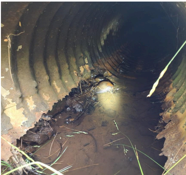
Figure 16: Example of a rusted culvert inspected during the 2025 field season (Culvert ID # 218).
